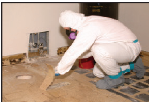
Prying up a section of flooring
