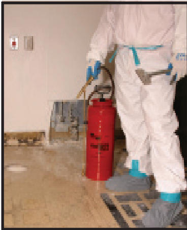
Using a tank sprayer to wet seams
