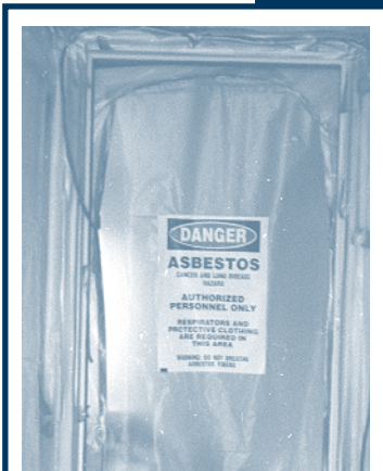
Containment Area Secure Entry Point
