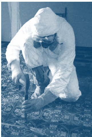
Cutting the Floor
