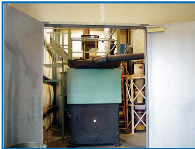
Talbot's Model C4 Warm Air Combustion Unit
