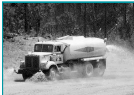
Using water or a chemical dust suppressant is one way to minimize dust emissions.
