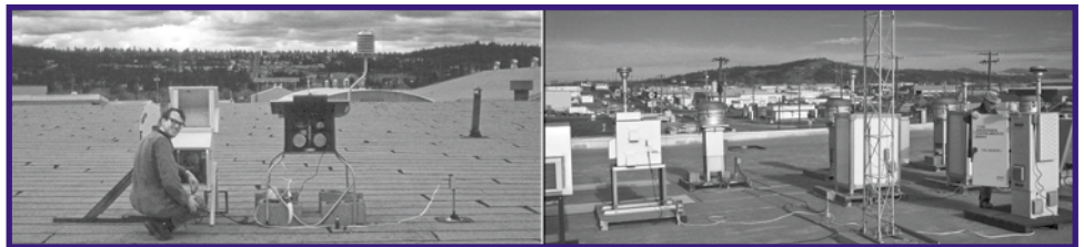
In 1969, there were a couple of air quality monitoring locations, including the one pictured above on the roof of the Crown Zellerbach warehouse, near Freya St. and Ferry Ave. The photo on the left is from 1969 and one the right is the site today. The current air monitoring network consists of nine sites, including new sites in Spokane Valley, Liberty Lake, Airway Heights, and Deer Park.
